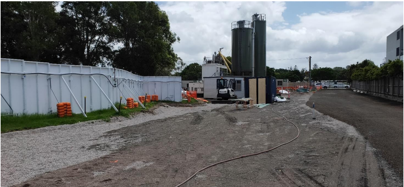
Photograph C.7 Mine Void Grouting operation
