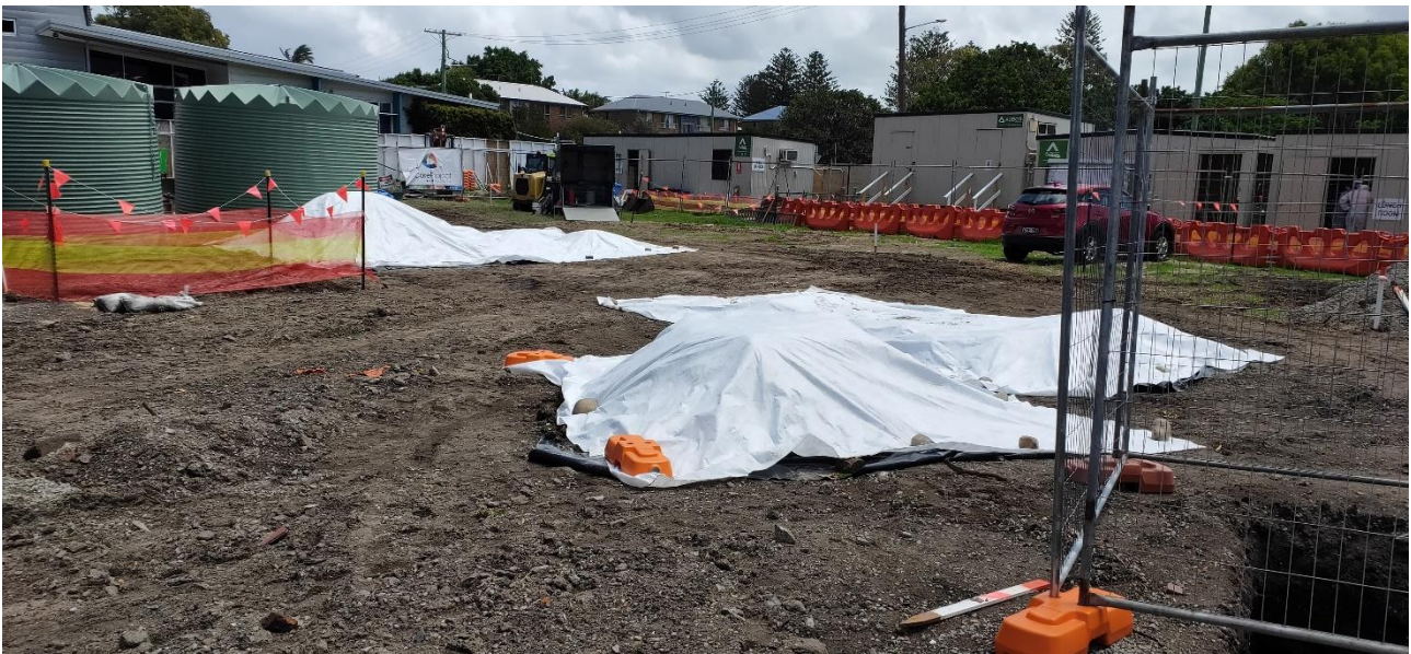
Photograph C.4 Excavated spoil material awaiting contamination testing and classification
